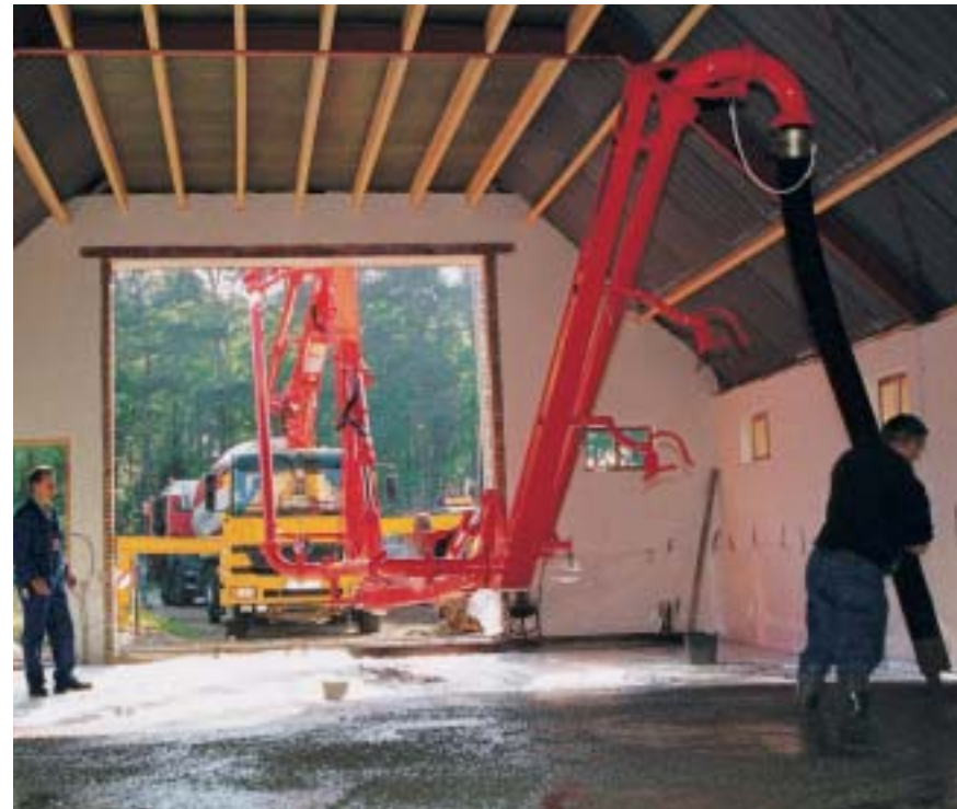
Surpasses all others for placing concrete in halls – thanks to low unfolding height and flexible Z-roll fold
